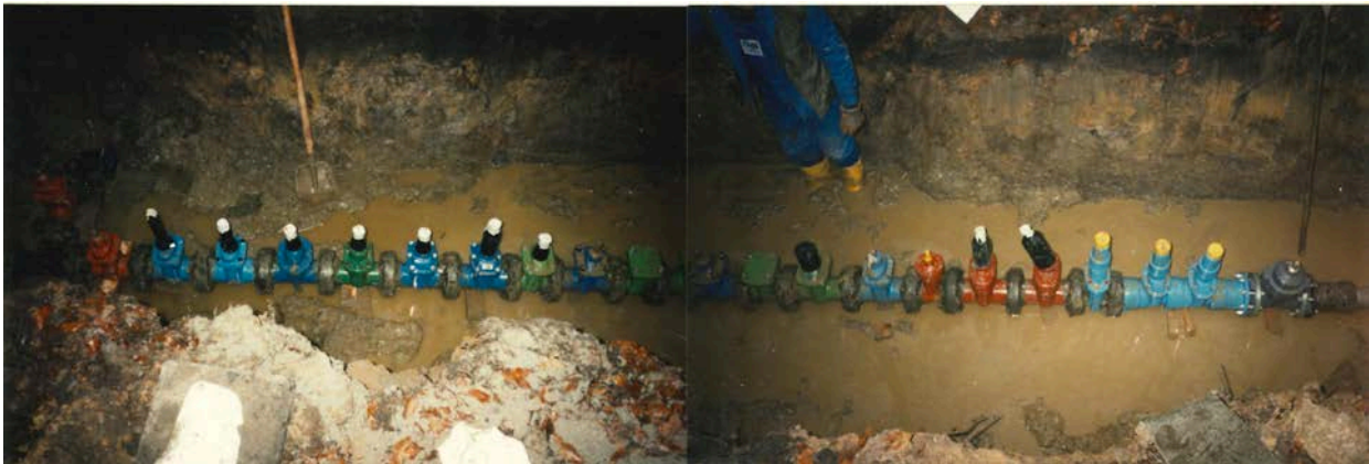
Test section consisting of 26 valves and fittings during installation in 1996
